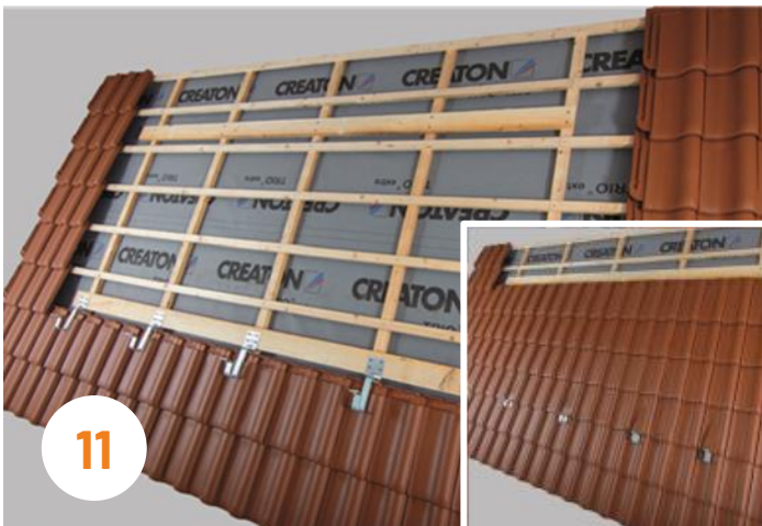
11 Screw the next wooden board and lay the tiles/roof tiles up to the lower edge of the wooden board..
