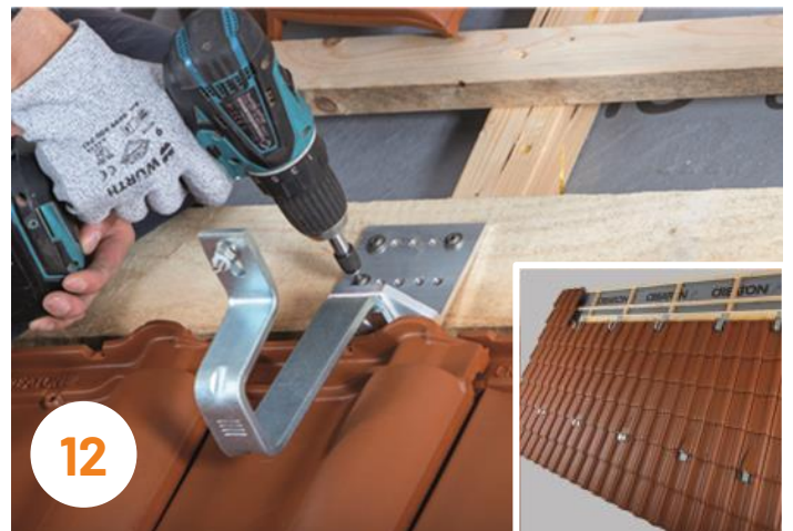
12 Fasten the next row of solar supports in the same way as previously shown with 4-4 pcs of screws in the corners.
