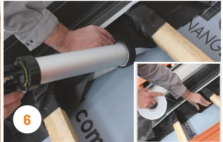
6 It can be attached to the membrane using either the swissporTON seam adhesive strip NKS or the CREATON special adhesive SKL.
