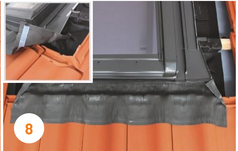
8 The abutment tape on the flashing frame is adapted to the profile of the tiles. The butyl adhesive tape attached to the underside is glued to the row of tiles underneath. The respective corners of the lead apron must be bent accordingly.
