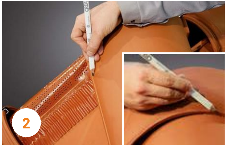
2 Position the last hip tile onto the edge and mark the line of the cut. Cut the hip tile to size along the mark using a disc cutter.
