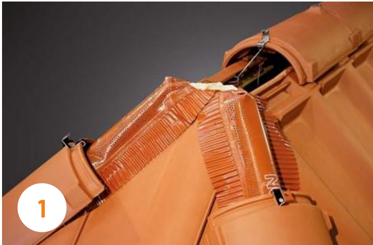
1 The apex of the hip is the cross-point where the hips meet with the ridge
