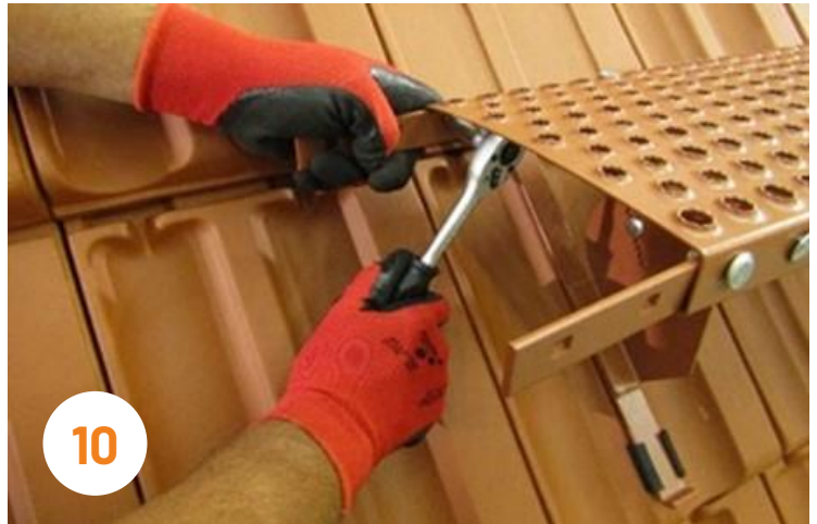
Use the walking grid assembly set if you want to make a continuous walking grid.
